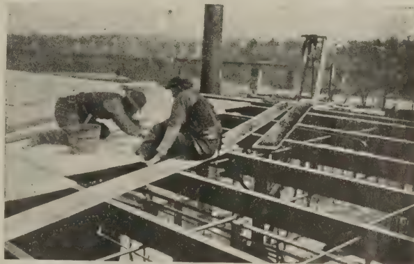
Roof construction—Steel channels and porous slabs
